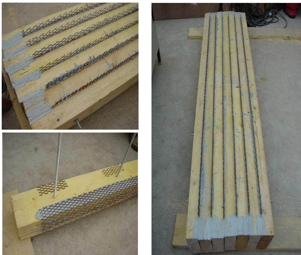
Figure 6. Preparation of connection of a composite slab
